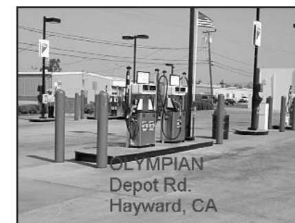
Olympian Cardlock on Depot Road in Hayward
